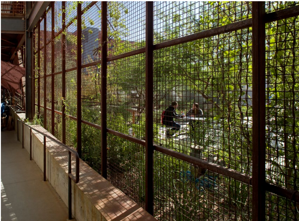
A Green Screen Cools the Building while Supporting Habitat
