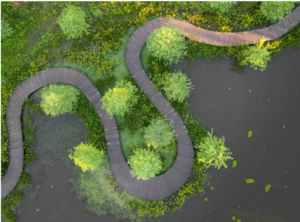
Wetlands Detain and Reuse Stormwater for Irrigation and Provide Habitat for Insects, Amphibians, and Birds. Courtesy Brandon Huttenlocher / Design Workshop Inc.
