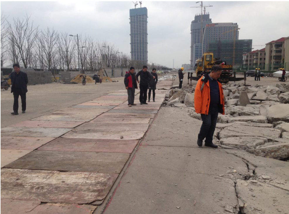
Photo of Construction Prior to Runway Transformation / Sasaki
